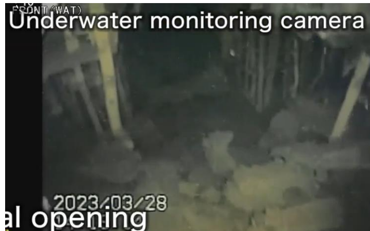
Figure 6-5: View of the pedestal opening.
