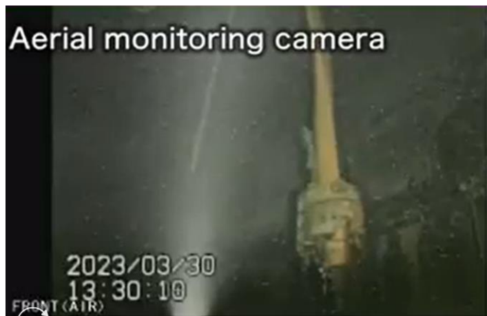
Figure 6-2: CRD housing hanging upside down under the RPV.
