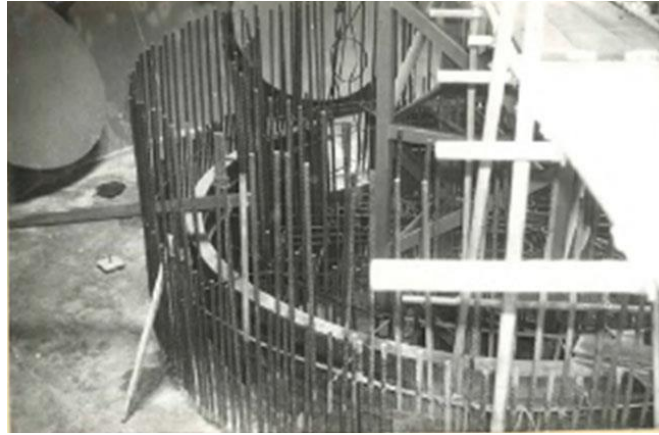
Figure 6-7: The inner skirt during construction.
