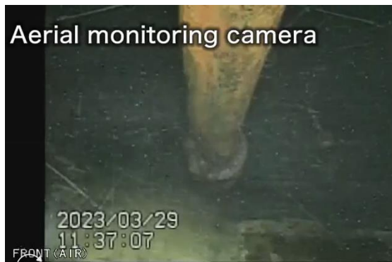
Figure 6-1: Dislocated CRD housing.
