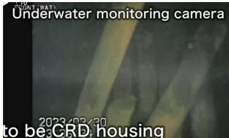
Figure 6-3: CRD housing buried in deposits and leaning on the pedestal wall.
