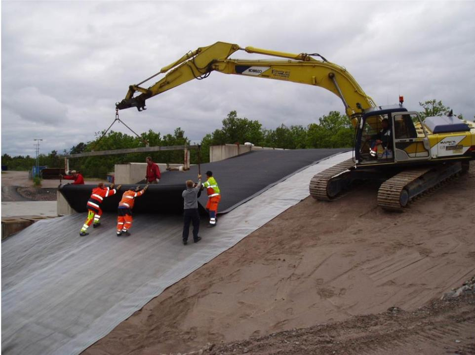
Figure 19. Construction of the final cover. Images from former disposal campaigns for MLA2 (2004). Image from former disposal campaign for MLA2 (2004).
