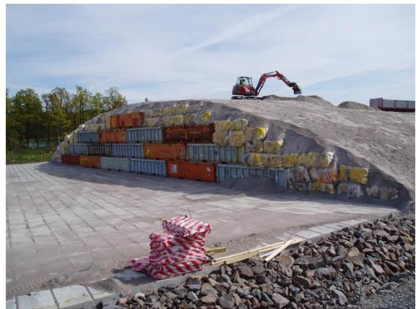
Figure 17. To the left: Each container is filled with stone flour in order to minimize air pockets and to create stability over time. To the right: Structure of landfill with a core of containers and garbage bales on top. Images from former disposal campaigns for MLA2 (2004).
