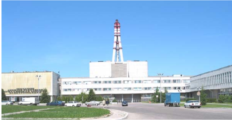
The Ignalina nuclear power plant in Lithuania
