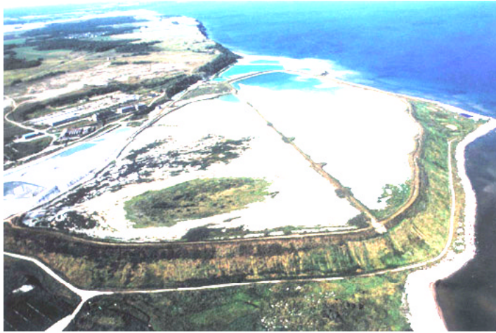
The Sillamäe site in 1996 before remedial actions were started. The steep dam wall and the undisturbed shoreline subject to erosion are clearly visible.
