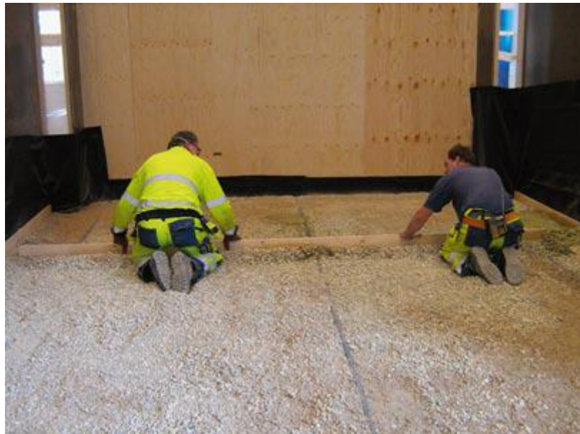
Figure 4_10. Preparation of the backfill foundation bed using Minelco granulate (SKB R-08-59).
