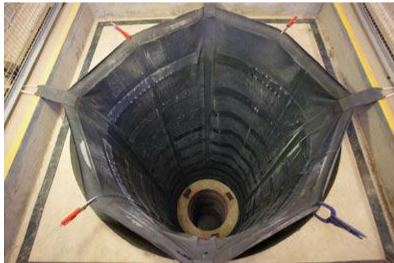
Figure 4_9. Rubber sheet for protecting buffer blocks from water inflows (SKB R-08-59).
