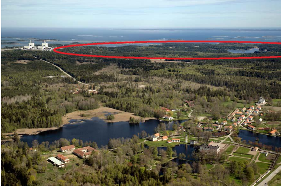
Figure 5: The Forsmark site, showing the nuclear power plant in the background, village in the foreground and with the approximate candidate area for the repository highlighted in red (adapted from Figure 1-4 of Lindborg, 2010).
