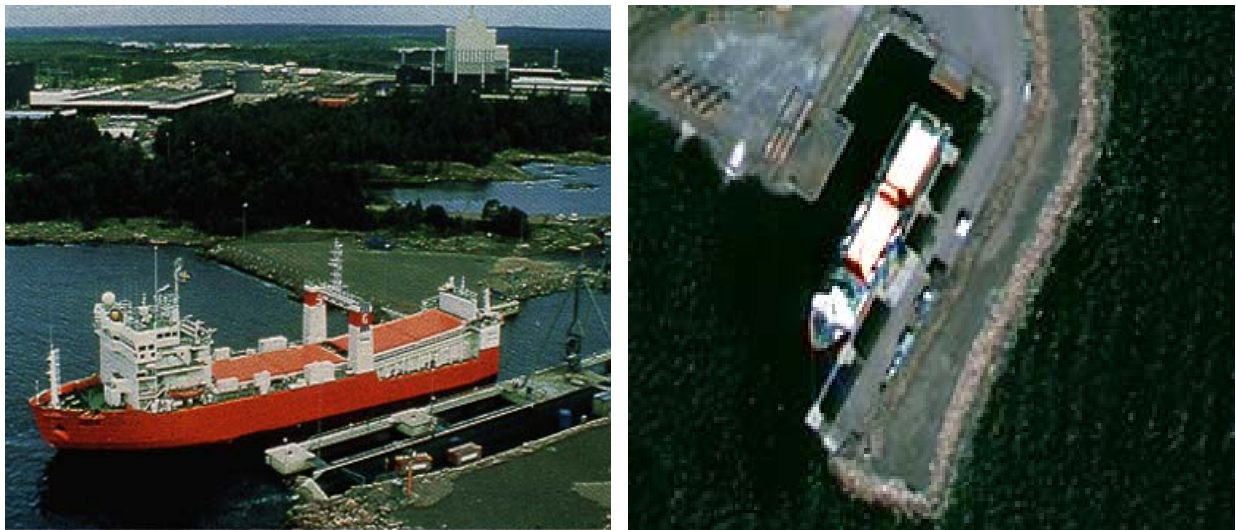
Figure 3: M/S Sigyn at the Oskarshamn Nuclear Power Station.
