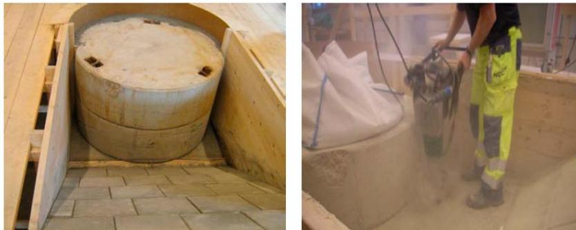
**Figure 2.10** Trials of backfilling the top of a deposition hole (from TR-10-16).
