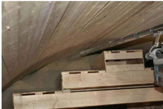
**Figure 2.12** Trial installation of backfill pellets (from TR-10-16).
