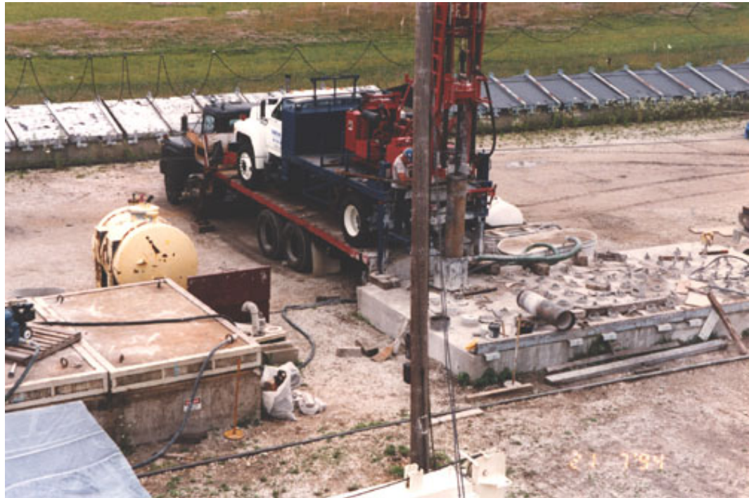
Figure 3-8 Core Drilling Rig on Flatbed Truck
