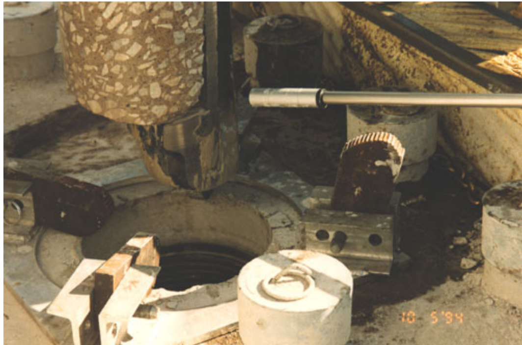
Figure 3-19 Core Drill Contact with Tube
