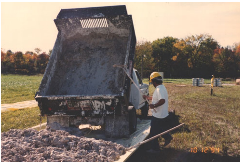
Figure 3-14 Dumping Concrete Fines
