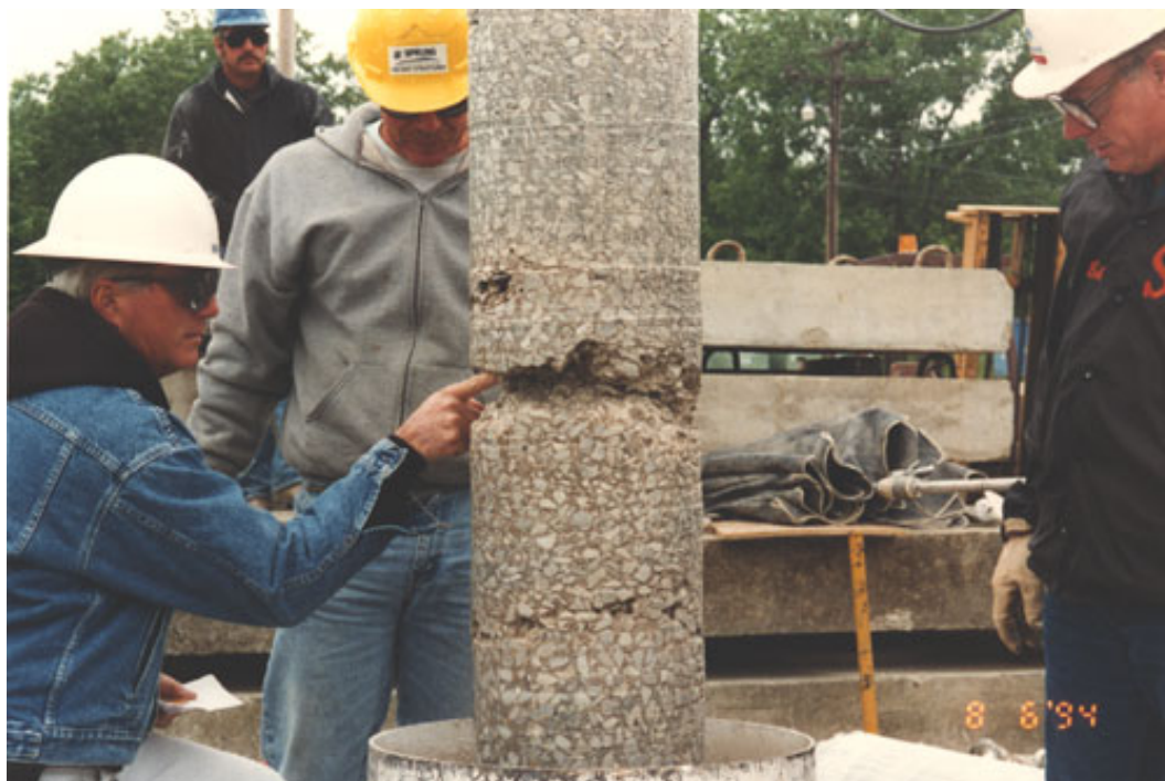
Figure 3-20 Voids in Concrete
