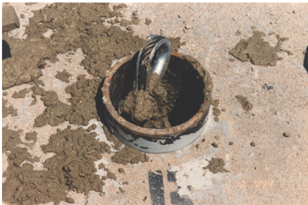
Figure 3-7 Lifting Eye Inserted in Tube
