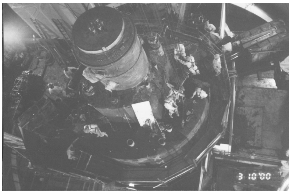
FIGURE 2.2 Removing the Biological Shield
